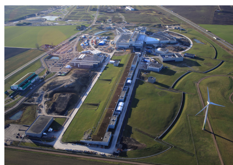
ESS, European Spallation Source in Lund, Sweden, is a multidisciplinary research centre built around the world's most powerful neutron source. TECHNIA is supporting ESS in creating a digital twin model that deals with design, building and production phases on an efficient and fully traceable basis. At the end of the usage phase, this also enables the ecologically responsible phase-out of the whole facility. Image: Perry Nordeng/ESS.
