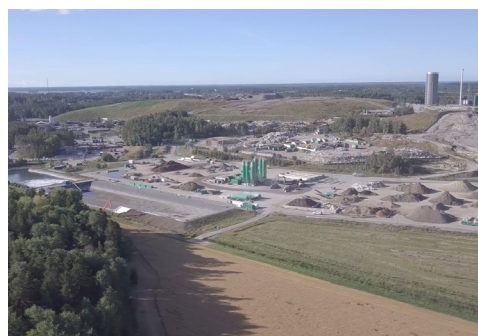
Sokigo has delivered its solutions TopoCad and CSM to environmental services group Ragn-Sells. The system enables the faster and more efficient design of Ragn-Sells' recycling plants, helping achieve better and safer recycling and waste management.
